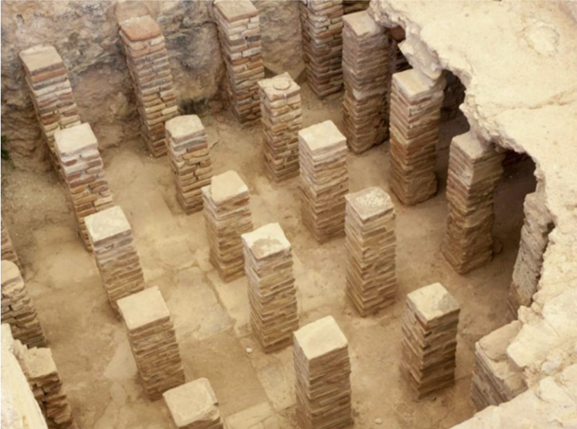
Fig. 2.1 Hypocaust heating system of antiquity
