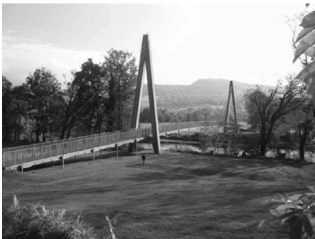
Figure 10.13 The Aberfeldy, Scotland foot bridge constructed from glass-fibre composites [11].
