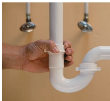
▲ Polyvinyl chloride (PVC) is used for pipes and plumbing fittings.
