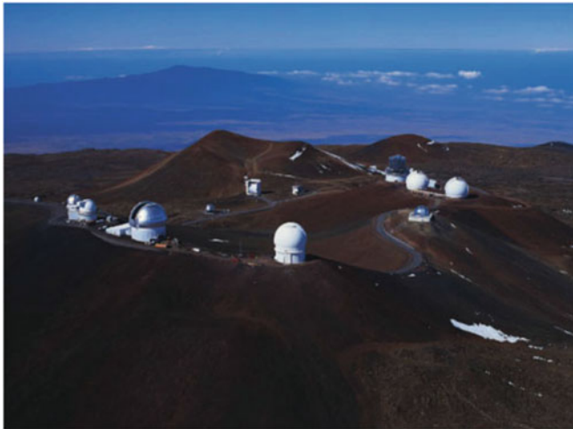
Fig. 5.9 The telescopes on Mauna Kea in Hawaii, USA. The two Keck telescopes (back right of image center) are twins; each has a mirror consisting of 36 segments (thickness only 7.5 cm) with a total diameter of 10 m. The segments are made of Zerodur (low thermal expansion). The weight of the glass is about 15 t; the mount is azimuthal. The total weight of the moving parts is about 300 t
