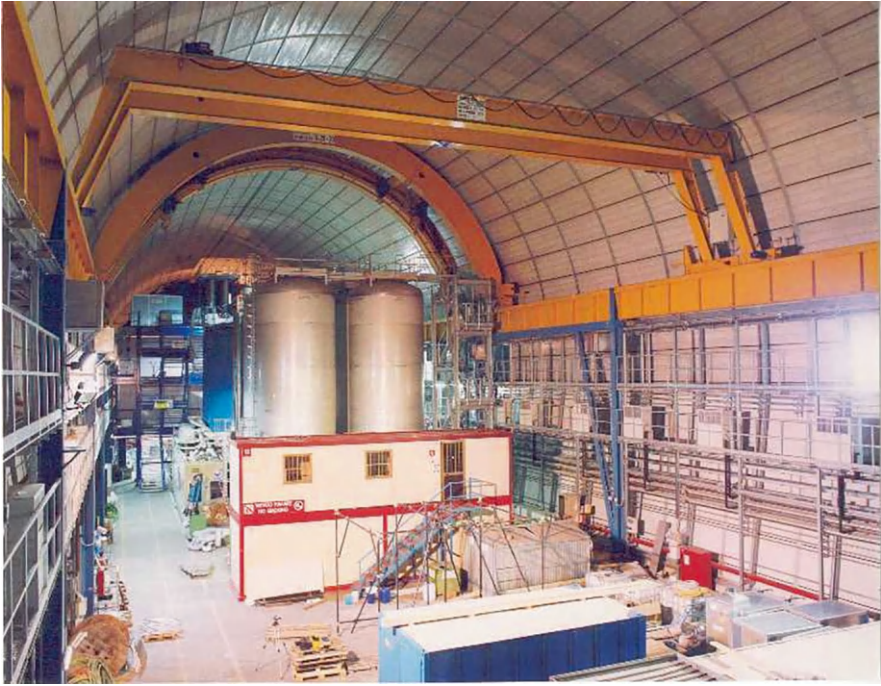
Fig. 5.10 General view of room C, with the storage area for pseudocumene visible in the foreground. The area contains our cylindrical containers designed to hold the pseudocumene. For safety, these containers are enclosed by a square containment wall capable of holding the entire volume of liquid in case of a rupture in one or more of the cylinders. The containment area is equipped with rapid fire-extinguishing systems and oxygen sensors. Cooling systems are installed. Above the containers to spray cold water onto the cylinders if their temperature rises for any reason. Additionally, fire-extinguishing systems are in place. Later, a blowdown system will also be installed (see later)
