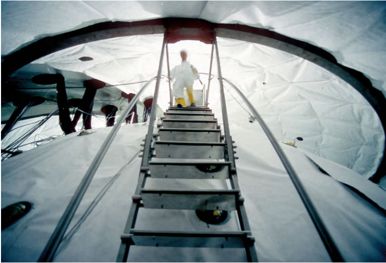
Fig. 6.15 The outer surface of the sphere and the inner walls of the Water Tank are covered with Tyvek. This covering is carefully designed to leave the photomultiplier sensors (eyes) exposed, allowing them to protrude through the Tyvek layer. The operator visible in the image is Paolo Lombardi
