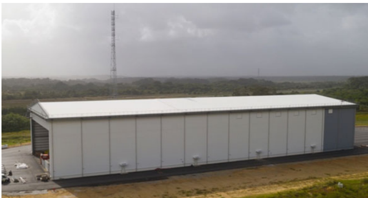
Fig. 2 Launcher assembly building (BAL)
