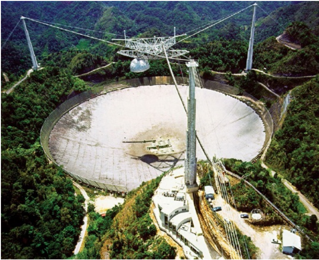
The semispherical radio dish of the Arecibo Observatory, 1,000 feet (305 meters) in diameter, nestled into the mountains of northwestern Puerto Rico. The platform hanging above the dish is a 900-ton structure that contains radio and radar transmitters, receivers, and support structures.
