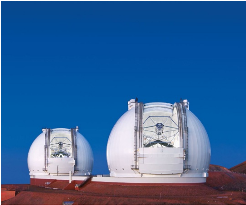
The twin telescopes at the Keck Observatory, near the summit of the extinct Mauna Kea volcano (elevation 13,600 feet [4,145 meters]) in Hawaii. Each telescope is 10 meters (33 feet) in diameter.
