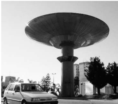
A water tower in the shape of a UFO was constructed in Varginha, Brazil, to commemorate the 1996 sighting.
