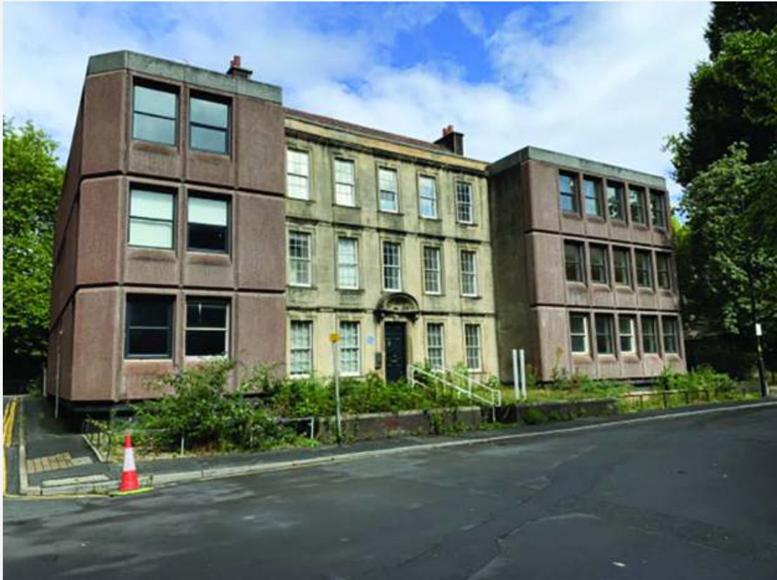
FIGURE 4.1 Redcross Street—From Dereliction to Designed Regeneration
