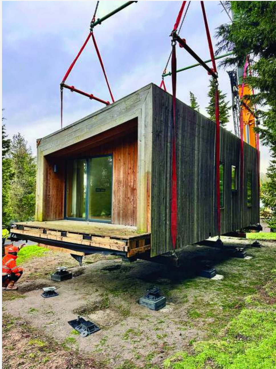
FIGURE 4.5 Precision-Manufactured Modules Craned into Position
