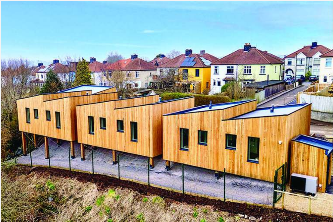
FIGURE 4.6 Agile's Low-Carbon, Timber-Framed Modular Homes in Operation
