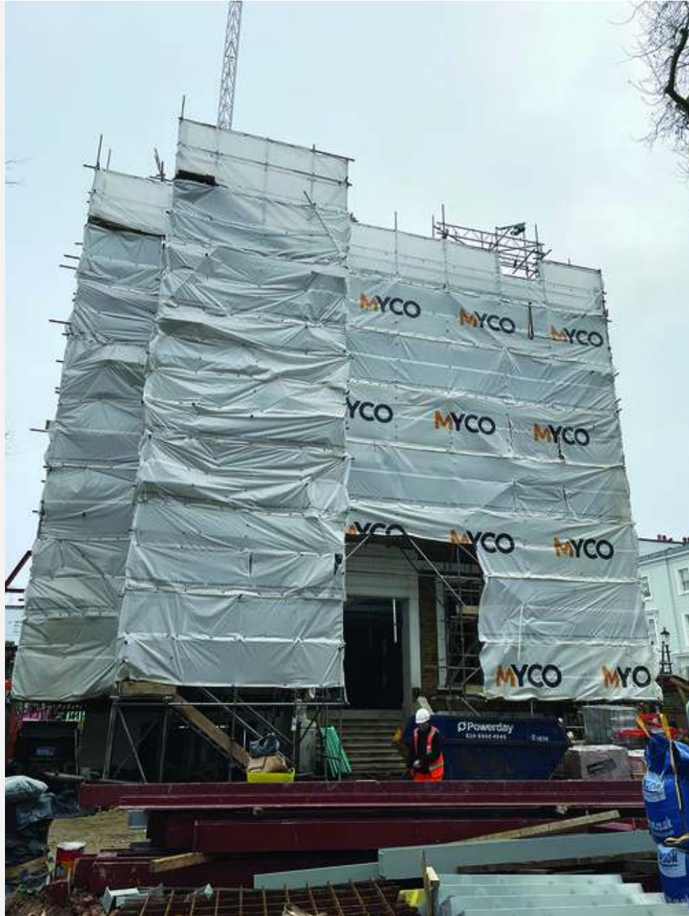
FIGURE 3.7 Atlantic House Approaching Completion (Final Stages of Refurbishment)
