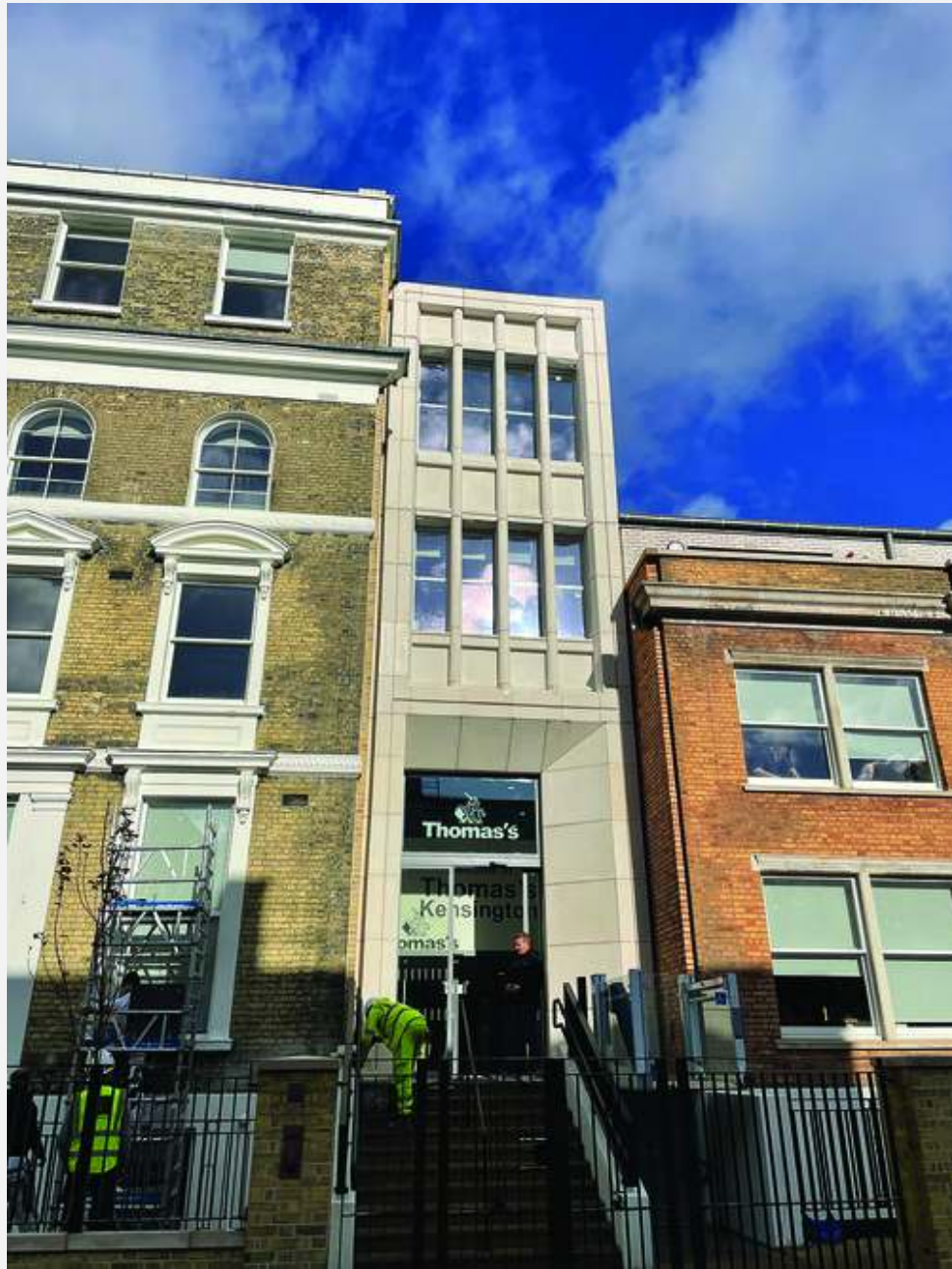
FIGURE 3.8 Completed Thomas London Day School, Kensington (Post-Refurbishment)
