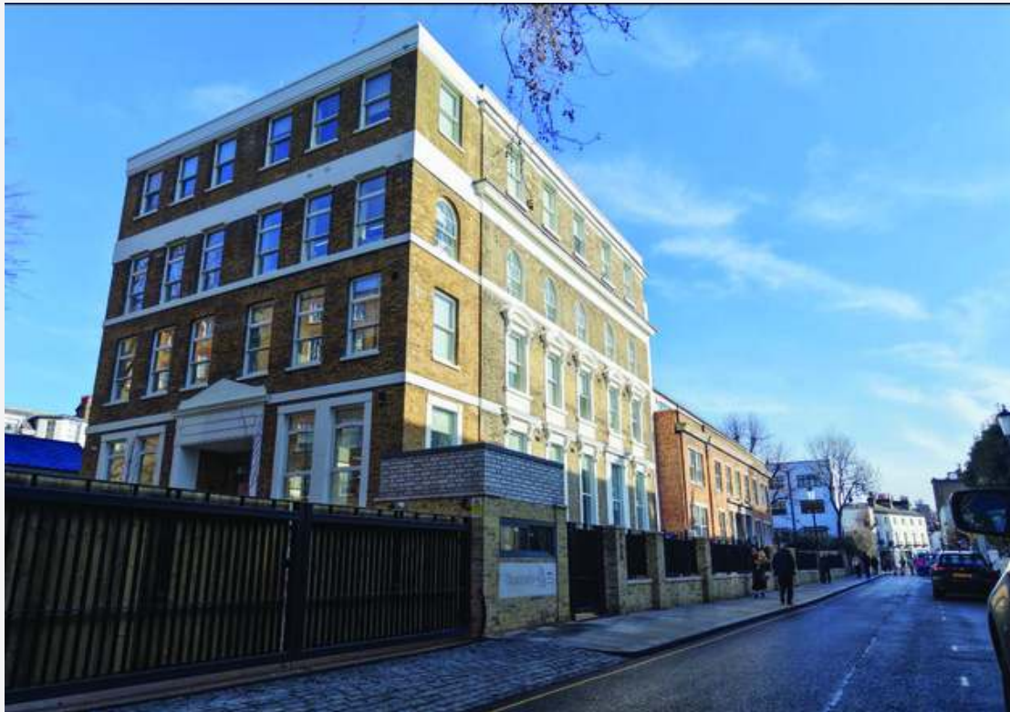
FIGURE 3.4 Atlantic House and Lytham House, Kensington (Pre-Acquisition)
