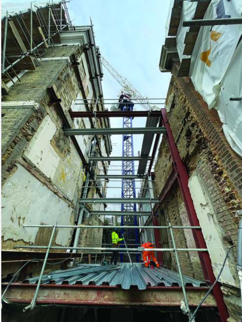
FIGURE 3.6 Refurbishment Works Underway at Atlantic House (Construction Phase)
