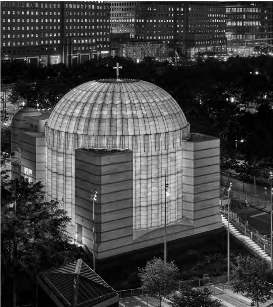
Figure 16.21 Santiago Calatrava, New York, St Nicholas Greek Orthodox Church at night, 2022, photograph. © Alan Karchmer/OTTO.
