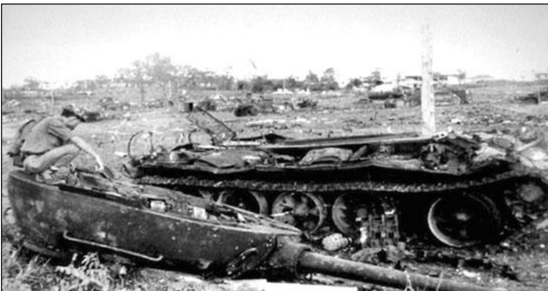
An ARVN soldier inspects a destroyed T-54. An internal explosion had blown away the turret. (US Army)
