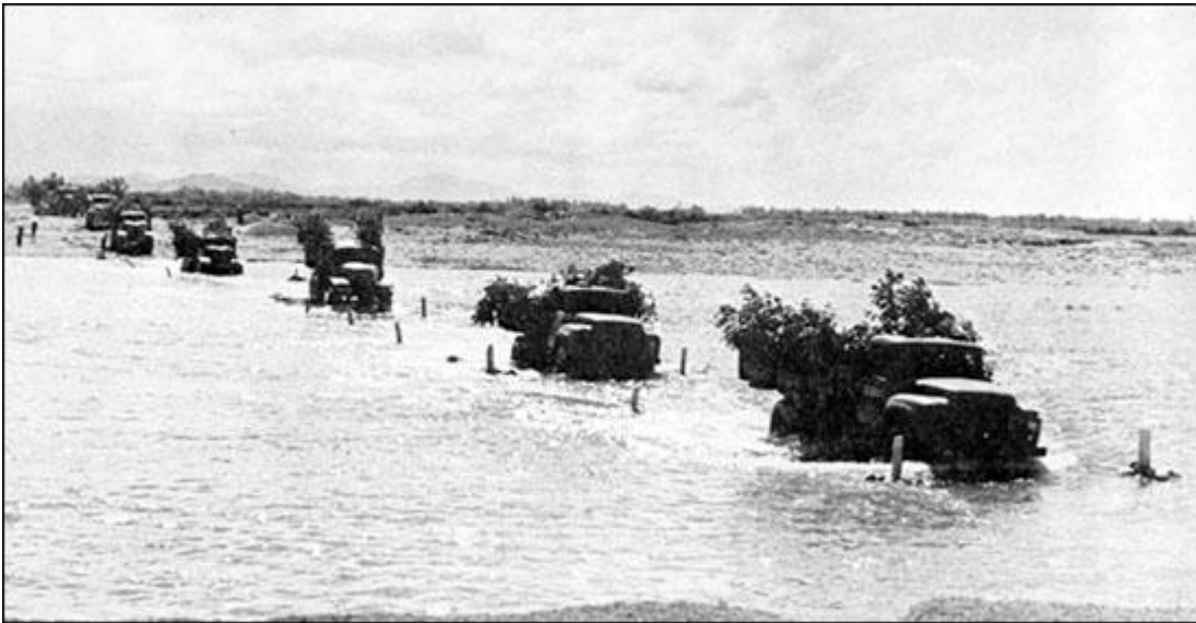
North Vietnamese engineering units became adept at quickly repairing and building new pontoon bridges to replace those destroyed by the airstrikes. One of the techniques used was to build submerged bridges to escape air detection. This column of ZIL-130 and ZIL-157 trucks crosses over one such submerged overpass. (PAVN)
