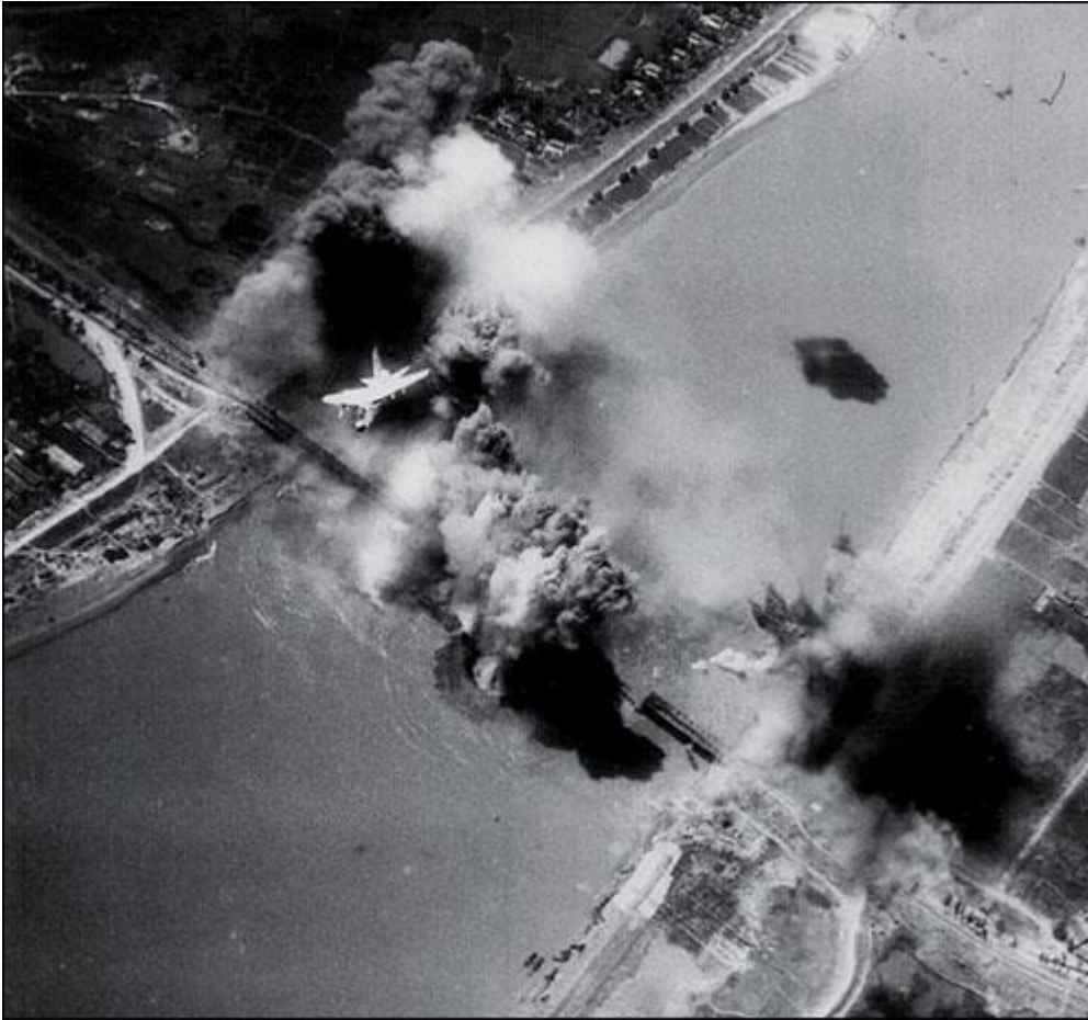
An A-7E Corsair II from the VA-195 pulls out from a bombing-run on the Hai Duong Railway Bridge on 10 May 1972. The American air attacks on the communication networks thwarted much of the North Vietnamese logistical efforts. (US Navy)
