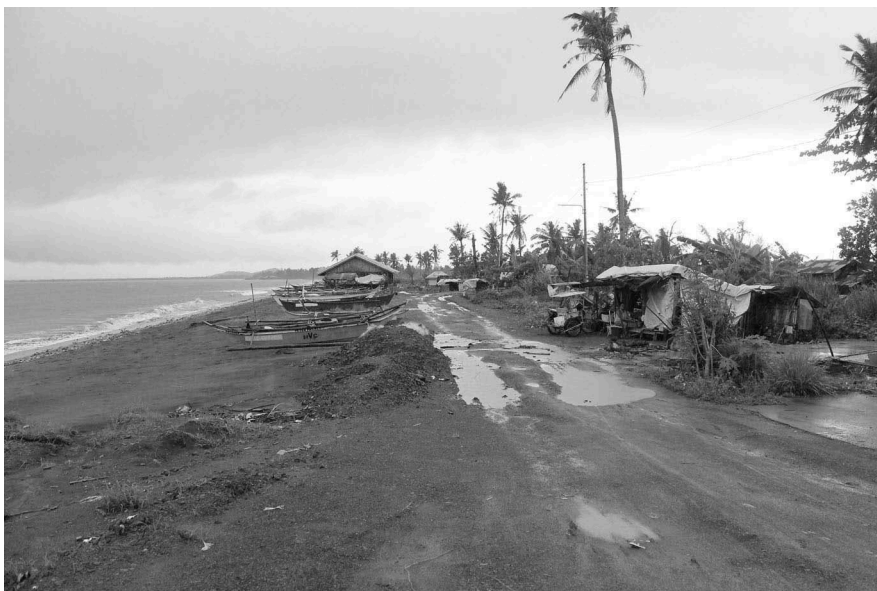
Figure 5.6 A bare shoreline in San Jose. This used to be a densely populated settlement before Yolanda struck.
