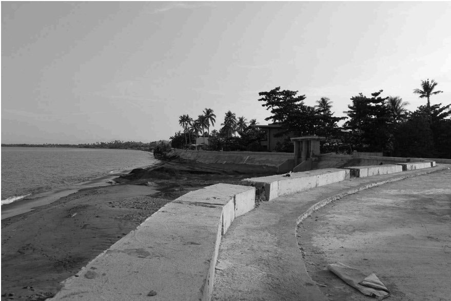
Figure 2.5 The concrete tide embankment
