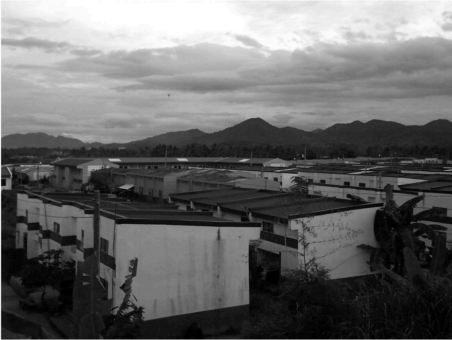
Figure 2.7 A view of Cawayanville, a resettlement site located in Barangay Cawayan, Tacloban North
