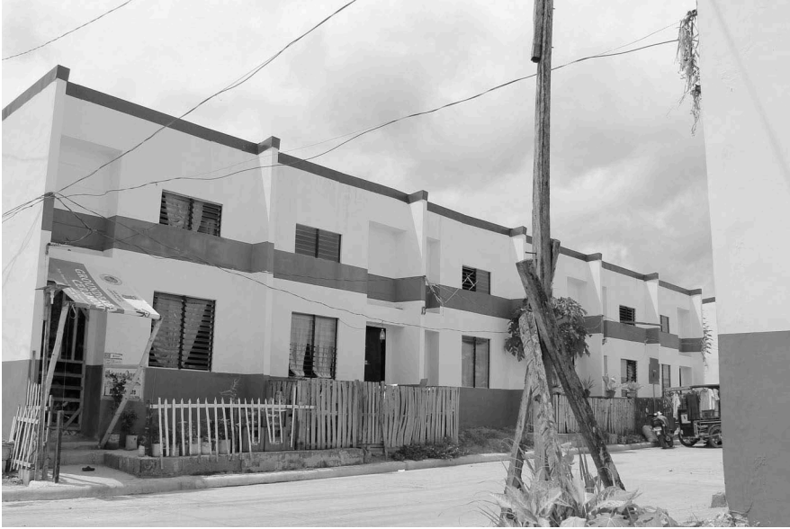
Figure 4.2 Rowhouses in Cawayanville
