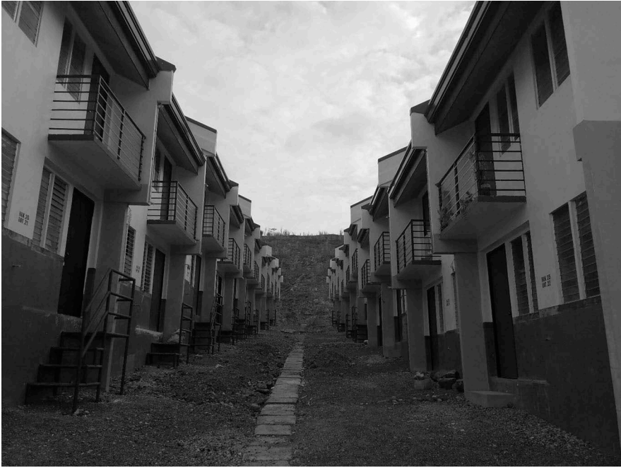
Figure 4.4 Two-storey housing at Pope Francis Village
